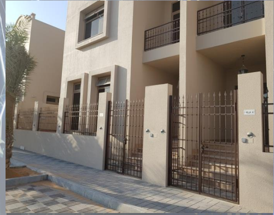
Handrails & Gates - Villa
