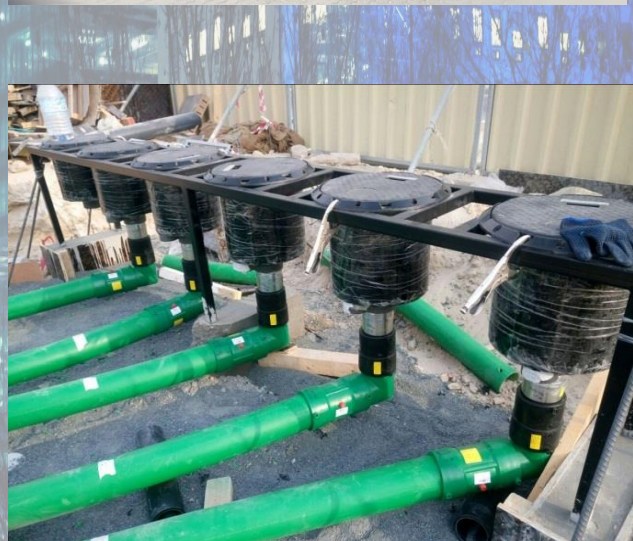
SPILL CONTAINERS (PETROL PUMP)
